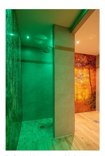
Two floor-level shower elements of the Fundo Primo series were installed in the new shower area. The factory-integrated slope ensures optimal drainage and thus reliably prevents water pooling on the floor.
